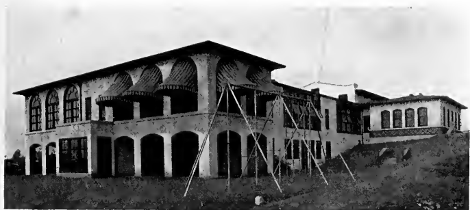
REAR VIEW OF CLEVELAND SCHOOL, OAKLAND John J. Donovan and Shafer & Wilde, Associate Architects
